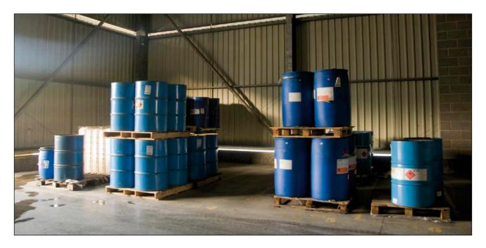
Figure 28 A purpose-built, bunded chemical drum store
