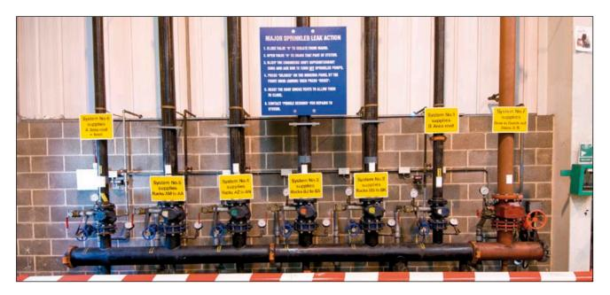
**Figure 41** Manifold for a sprinkler system
