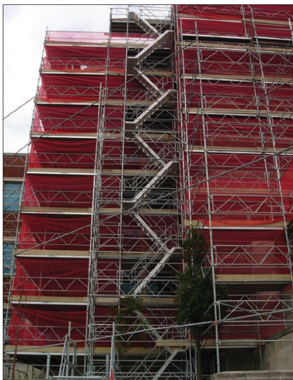
Figure 3 Stair towers provide good access. Make sure they are properly secured and erected (image courtesy of Turner Access)
