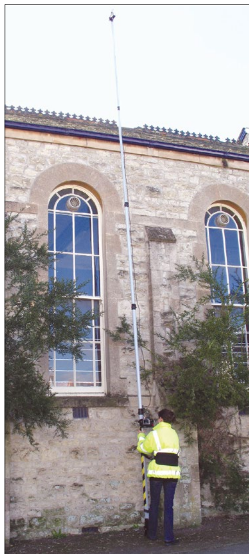
Figure 10 Remote inspection mast with hand-held lightweight CCTV system (image courtesy of Survey Support Ltd)
