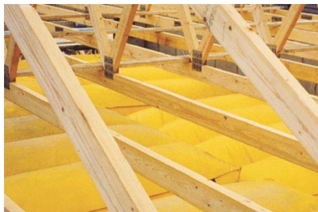
Figure 14(b) Airbags being used as a fall mitigation measure during roof work (image courtesy of Airtek Safety Products Ltd)
