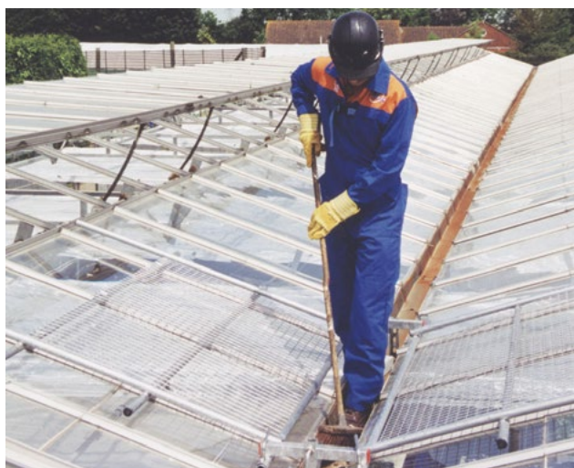
Figure 12 Valley walker used during gutter cleaning. This provides a protective mesh covering to either side of the operative, which moves progressively along the roof as the worker moves forward. The protective covering eliminates the risk of a fall through the fragile material (image courtesy of Safesite Limited)
