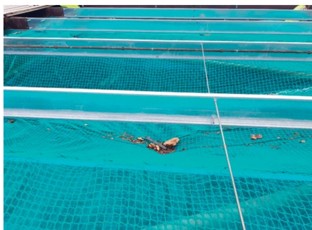
Figure 7 Debris netting used in addition to safety netting may enable work to be carried out safely below roof workers (Image courtesy of Highersafe (North East) Ltd)
