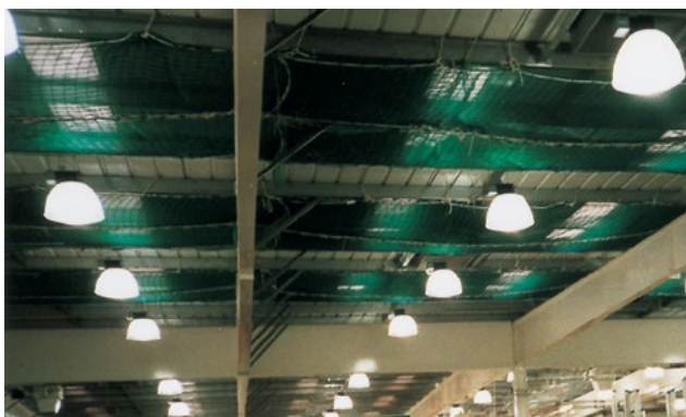
Figure 28 Safety netting used to minimise the distance and consequences of a fall for roof lights during roof works
