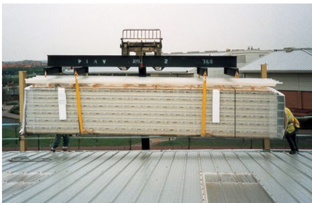
Figure 31 (above) Delivering sheets to roof level onto the completed load-bearing section and behind the leading edge (note that the roof lights include mesh protection and are non-fragile)
