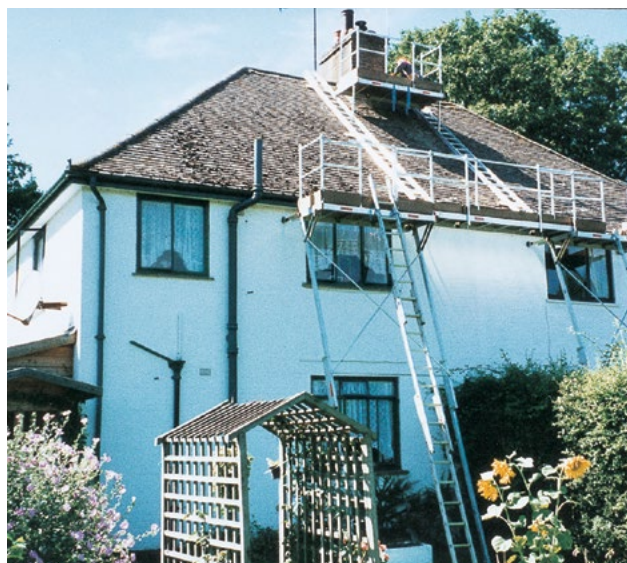
Figure 25 Proprietary system for access to roof and chimney
