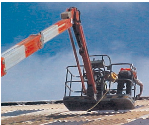
Figure 15 A mobile elevating work platform being used to replace a roof sheet
